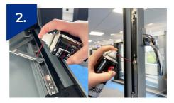
Add a small amount of lubricant at each pivot point and locking part\*
