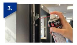
Lubricate moving parts of the lock mechanism using a suitable 3 in 1 light machine oil, wiping away any excess
