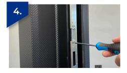
Check the tightness and security of all fixings, tightening as required
