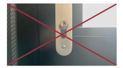
Do not routinely lubricate lock cylinder\*
