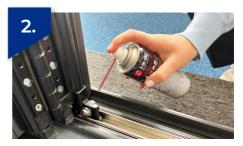
Lubricate the wheels as required using a suitable 3 in 1 light machine oil, wiping away any excess
