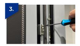
Check the tightness and security of rail & keeps
