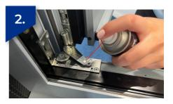
Follow steps 1 to 4 of the window hardware maintenance instructions but remember to lubricate the additional locking and hinge points that are present on a tilt and turn window including along the top and bottom of the window
