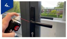
Use a light machine oil on moving handle parts, but not the lock cylinder
