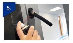
Use a light machine oil on moving handle parts, but not the lock
